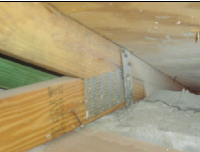
Roof to wall attachment
