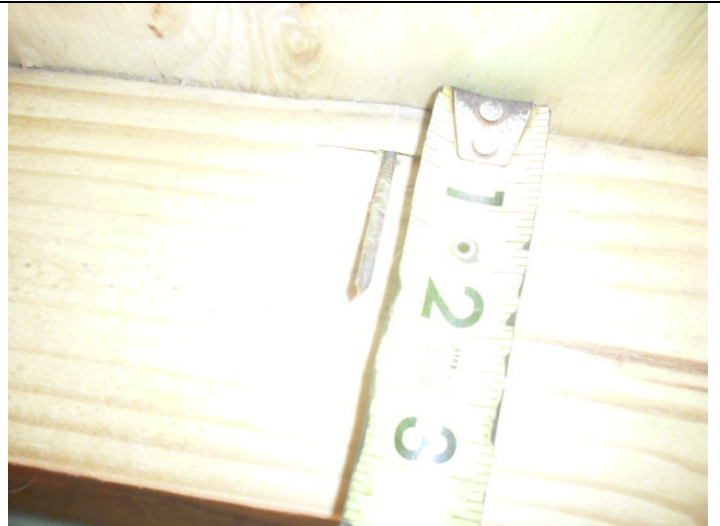
Roof deck attachment
