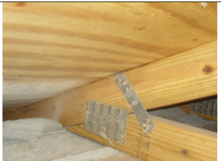
Roof to wall attachment
