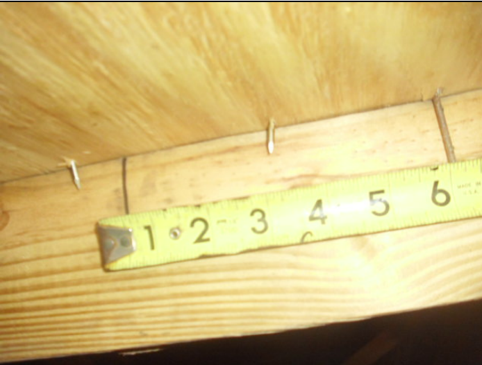
Roof deck attachment
